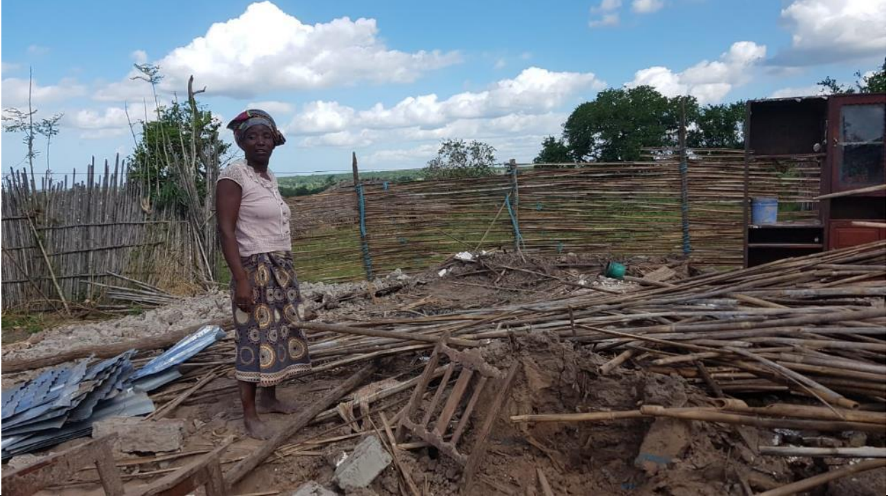
Over 370 Houses like this were destroyed
