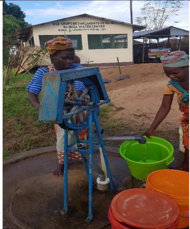
The Rope pump in front of the SMART centres is one of the few pumps still working in Bilibiza and over 200 people collect water every day.
