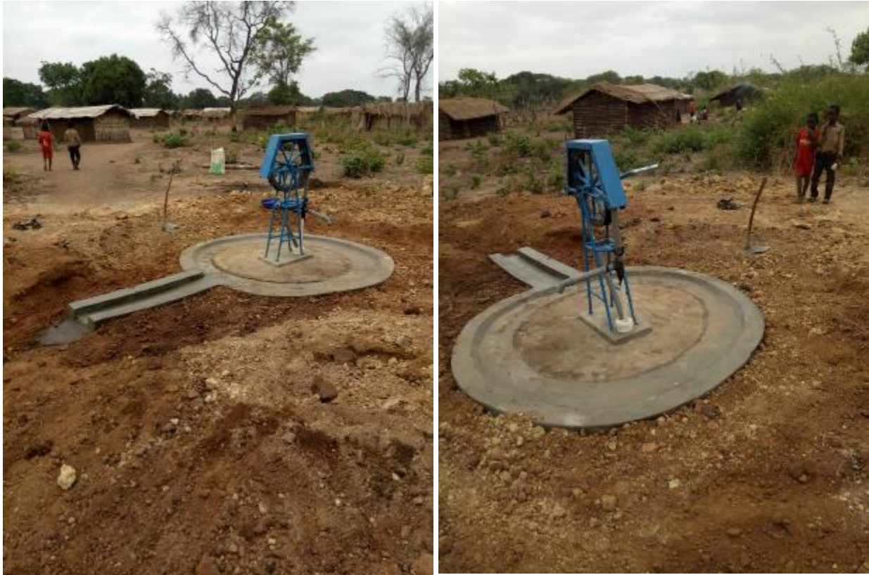
Picture 5: Second drilled tube-well in Balama District, Impiri Locality within the resettlement camp.
